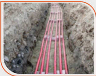
» FO cable laying & termination.
